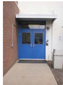
New main entrance door
