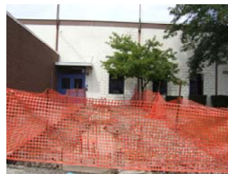
Phase III underway —main entrance
